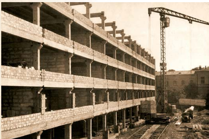
At a construction site of a new building for training
